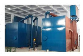
The main advantage of ZW gravity valveless filter is that it does not need to use large gate valve and operates automatically; The main disadvantage is that the filter material is in a closed pool, which is more difficult to remove the dirt on the surface of the filter layer that is difficult to wash for "sanding".
